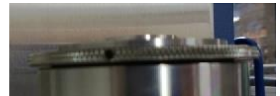
Bottom Plate Installed
